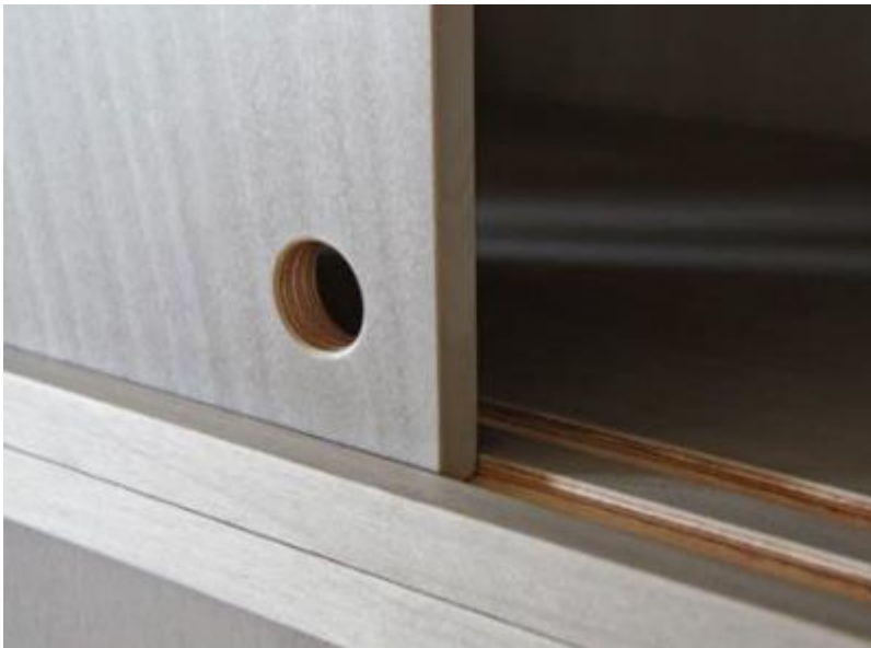
Traditional method grooves or insert laths
