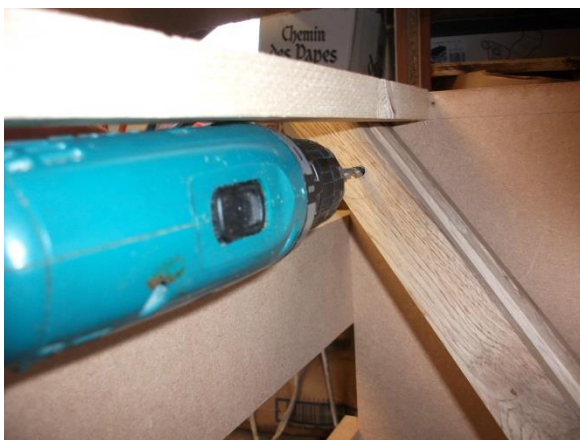
Image 64 Drilling legs for fixing bolt
