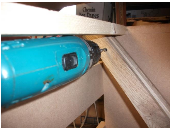
Image 64 Drilling legs for fixing bolt
