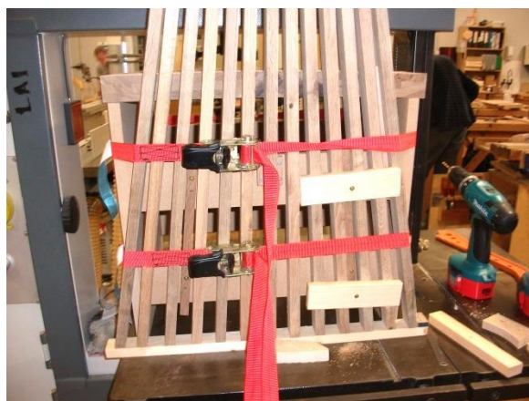
Image 47 Baton screw fitted in place
