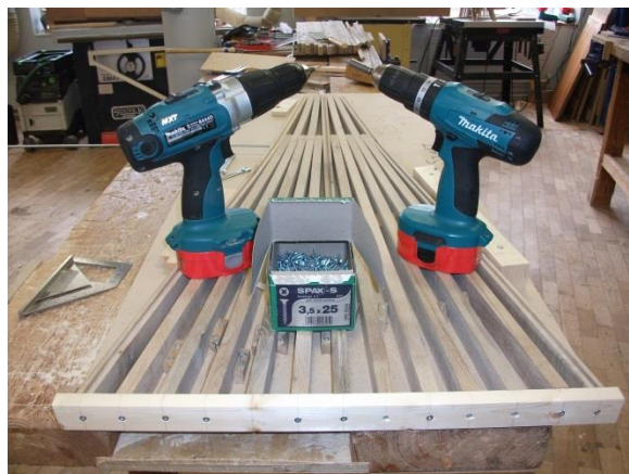
Image 43 Baton screw fitted in place
