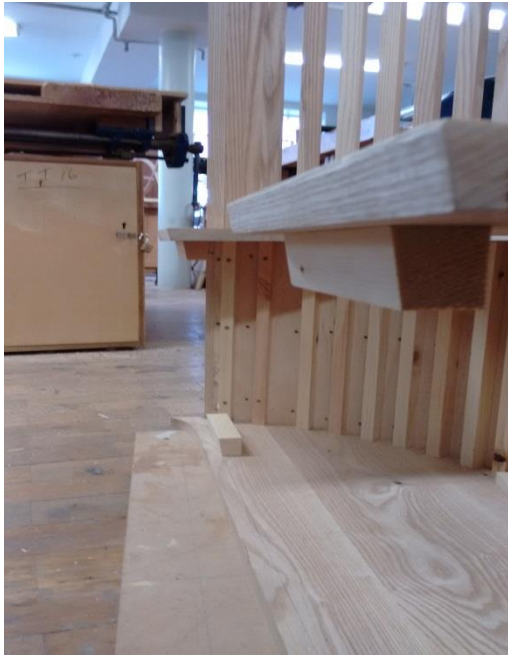
Fig. 95 Timber brackets fitted to seat.
